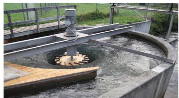
Fig. 1. A gravitation water vortex plant with a Zotlöterer turbine near Ober-Grafendorf, Austria.
