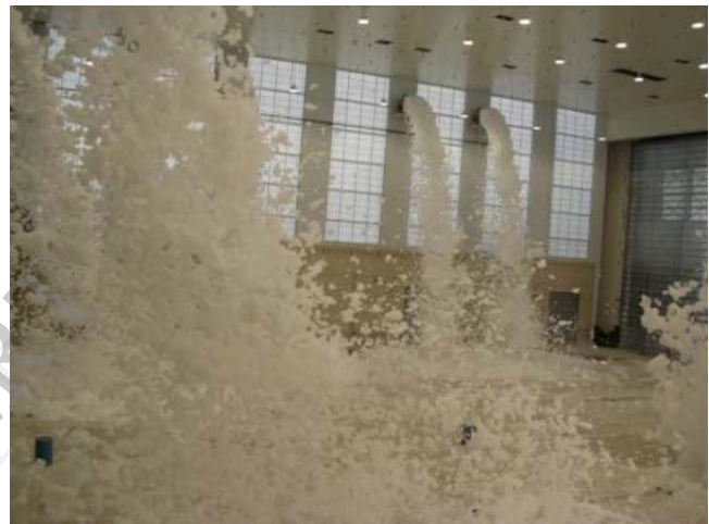
Figure 2. Operation of Deluge system
