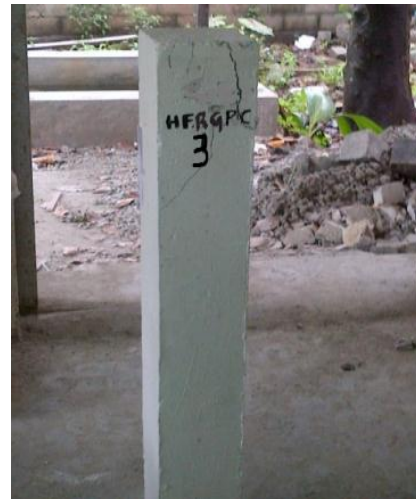
Fig 10 HFRGPC3 column after testing
