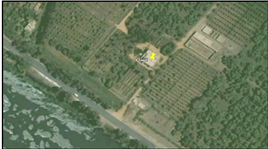
photo. (1) General location of North Giza power station
