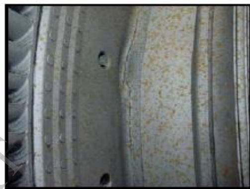
Fig. 1 Photo showing T.F. cracking in disc radii and balance hole (3)
