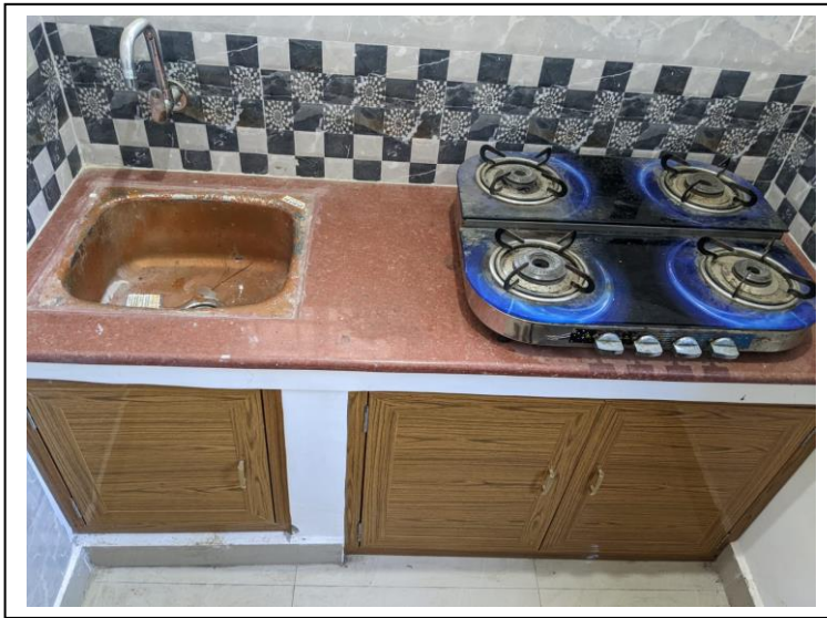
Figure 5 Kitchen platform and bottom storage with PVC shutters
