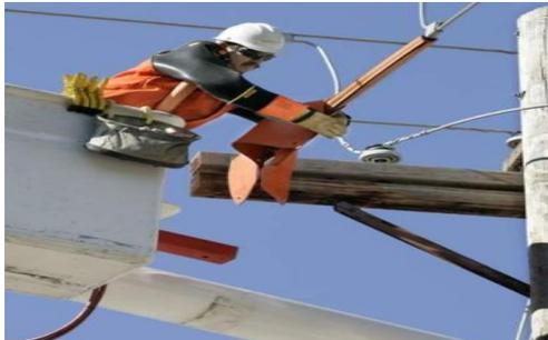
Fig. 2. Live line maintenance using insulating or rubber gloves
