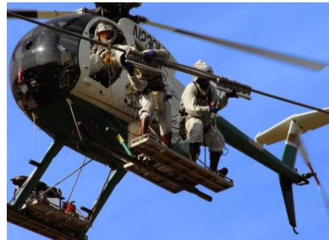
Fig. 4. Live line maintenance using helicopter platform
