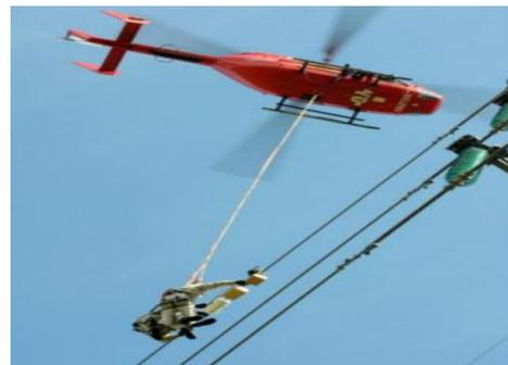
Fig. 5. Live line maintenance using helicopter sling
