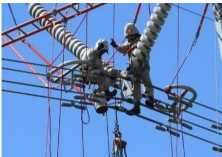
Fig. 3. Live line maintenance using bare hand
