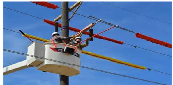
Fig.1. Live line maintenance using hot stick
