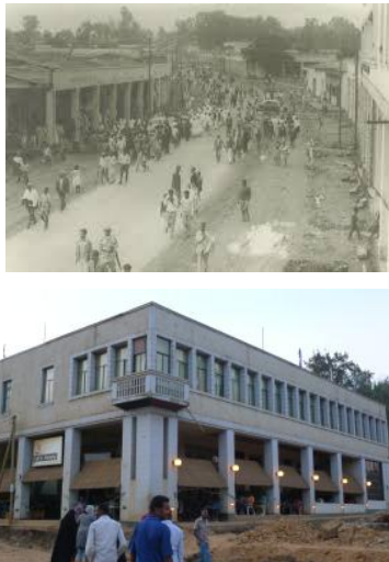
Fig 1. Existing Old Brick Buildings in Jimma town
