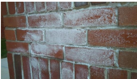
Fig 3. Effect Efflorescence
