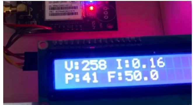
Fig.7 The LCD display showing real-time readings of the electrical parameters when the load is connected, and its range is below the threshold limits.
