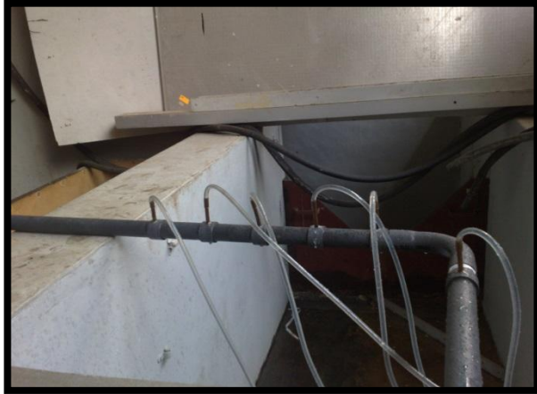
Fig 3.1 Copper pipes are reverted into PVC pipes
