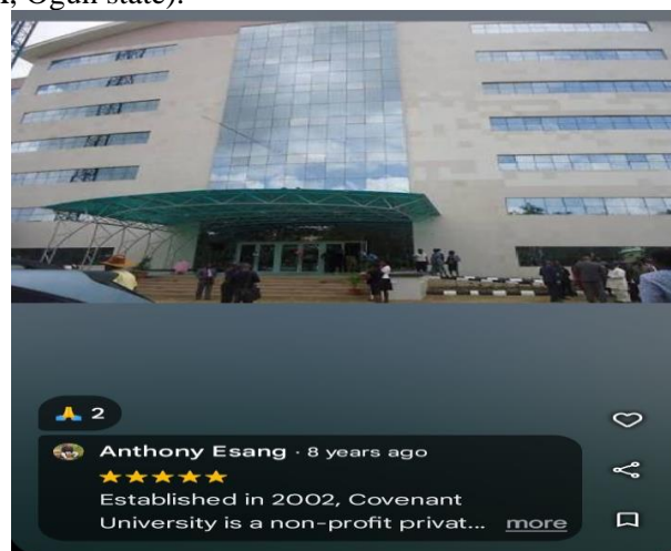
Plate 5. Location for sand sample chemical analysis.
