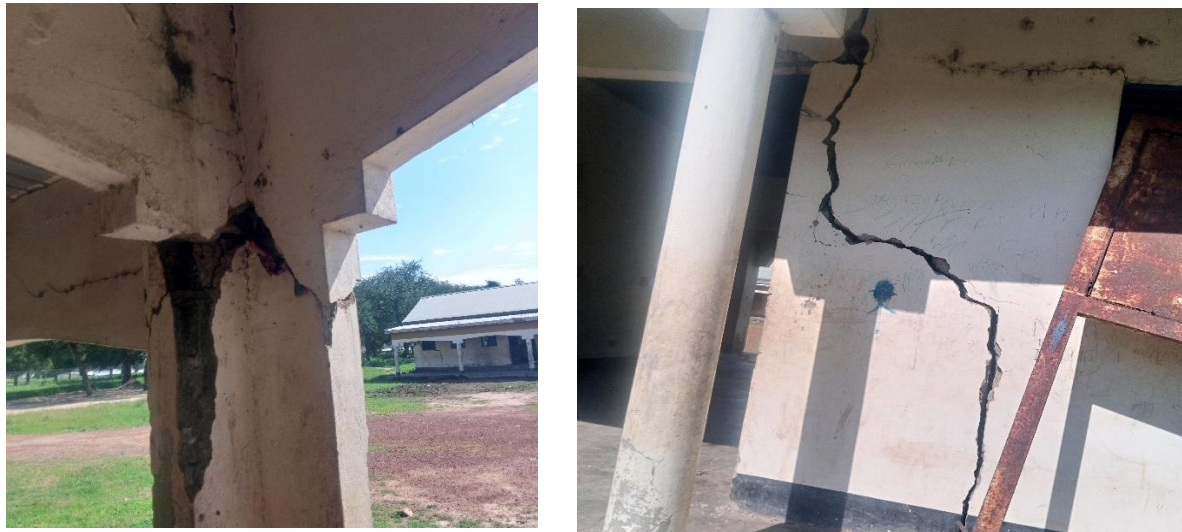
Fig 1.4 Sample of structures build on black cotton soil due to foundations failure.
