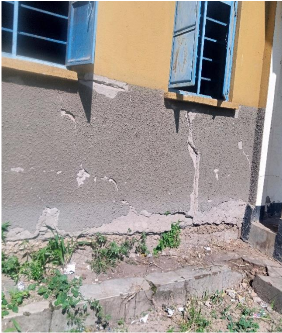
Figure 1.1 A typically examples of structural damage on black cotton soil in Juba, South Sudan
