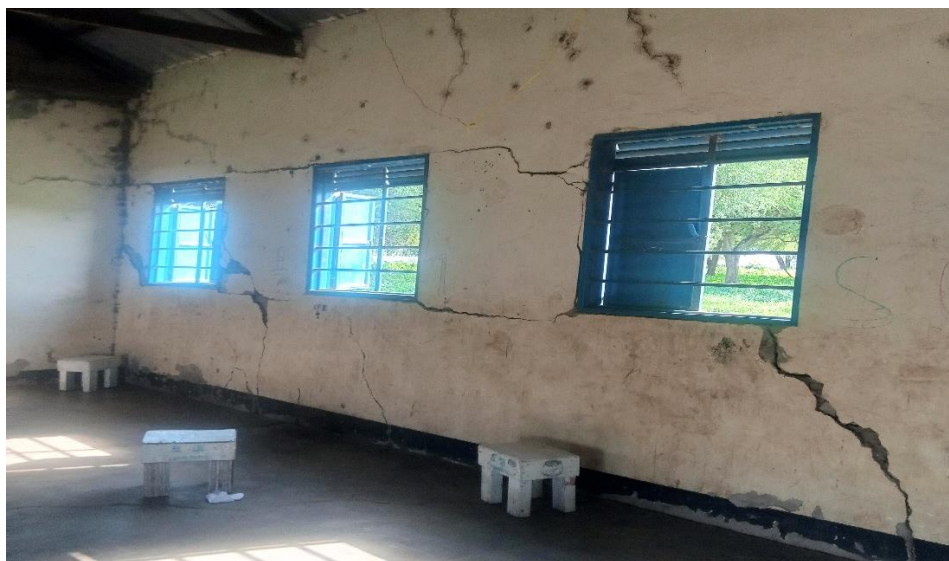
Fig 1.5 Several cracks on building resulting from uneven settlement
