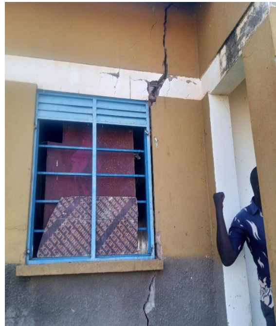
Figure 1.1 A typically examples of structural damage on black cotton soil in Juba, South Sudan
