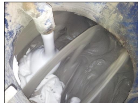
(a) Mixing of foam to mortar
