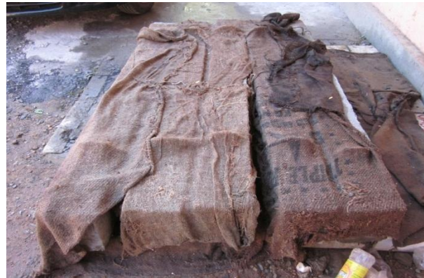
Fig. 3.17 Curing of Beam Specimens
