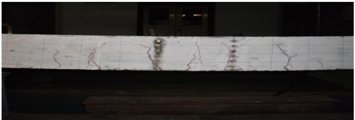
Fig. 4.37 Crack Pattern of R 6 Beam under Flexure
