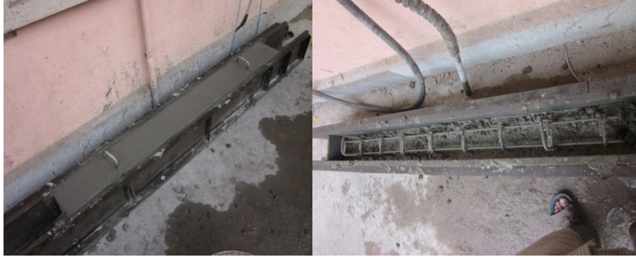
Fig. 3.16 Casting of Beam Specimens
