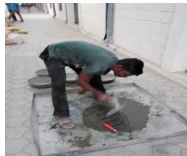
Fig. 1. Mixing of Concrete
