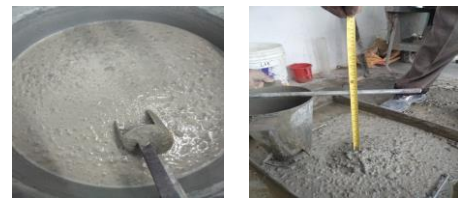
Fig-3: Mixing & slump test of concrete
