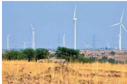
Figure 1: Wind Power Plant
