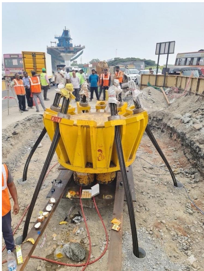
Fig 3. Initial Pile load test.Anchor Pull out method
