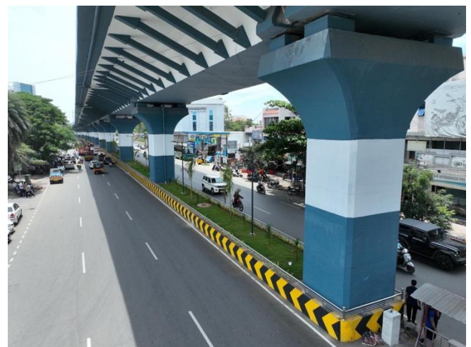
Fig 20 Pier Protection Wall with SS Railings
