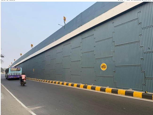
Fig 10. RE wall for Ramp
