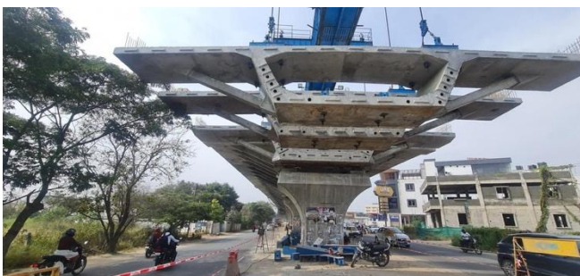
Fig 6. Segmented Box Girder.
