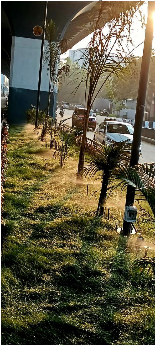
Fig 41. Sprinkler Irrigation in At-Grade Level
