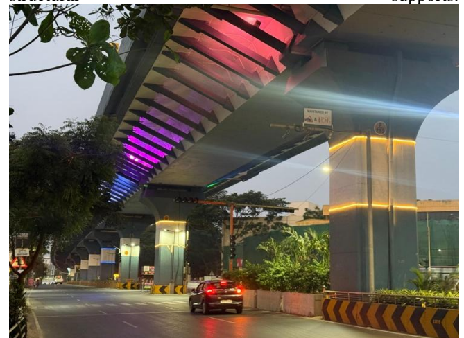
Fig 47. Strip lighting over Pier at Junction
