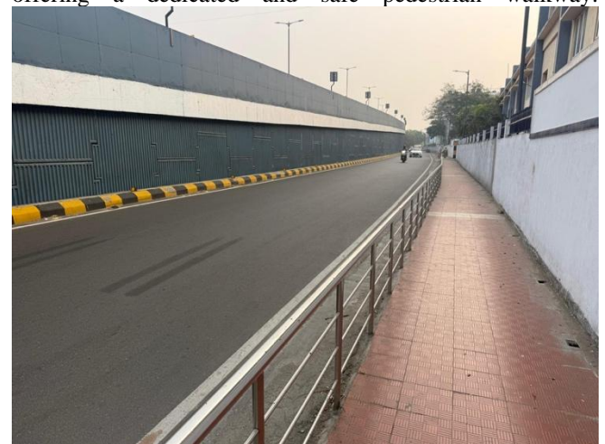
Fig 52. Foot Path with Hand Rails over Drain
