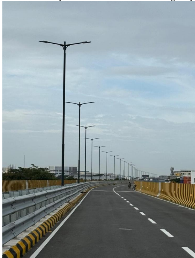
Fig 44. Lighting at elevated Level
