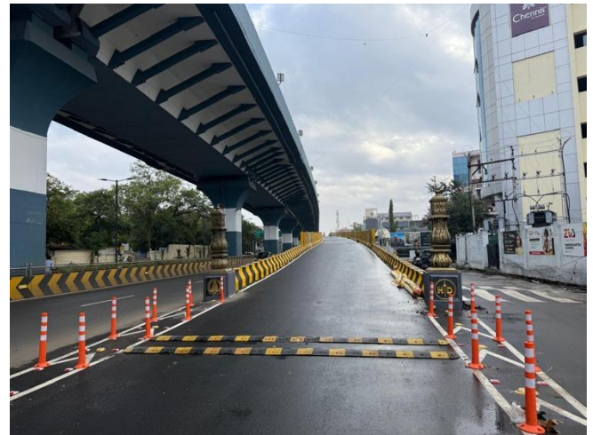
Fig 19. Temporary Rubber Speed breaker.
