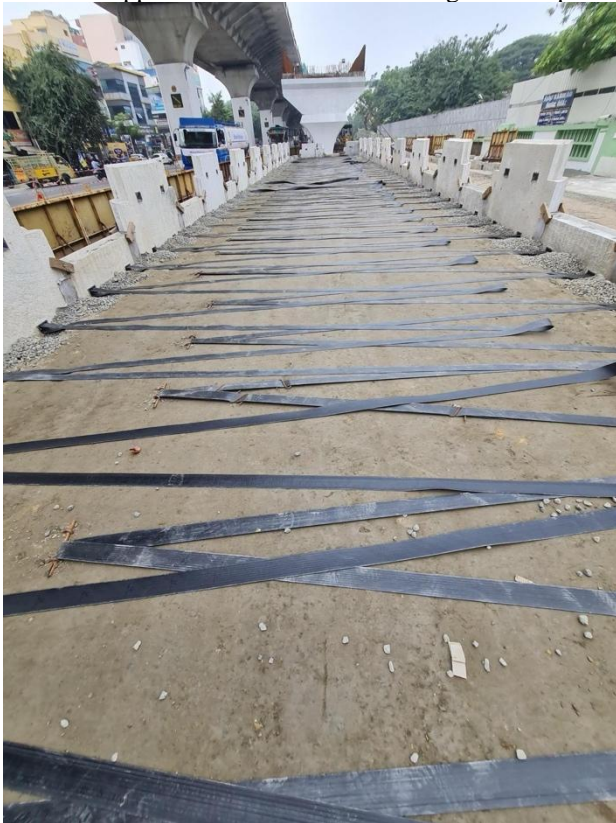
Fig.9. Geo Strips in RE Wall
