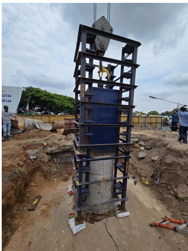
Fig 4. Dynamic Pile Load Test
