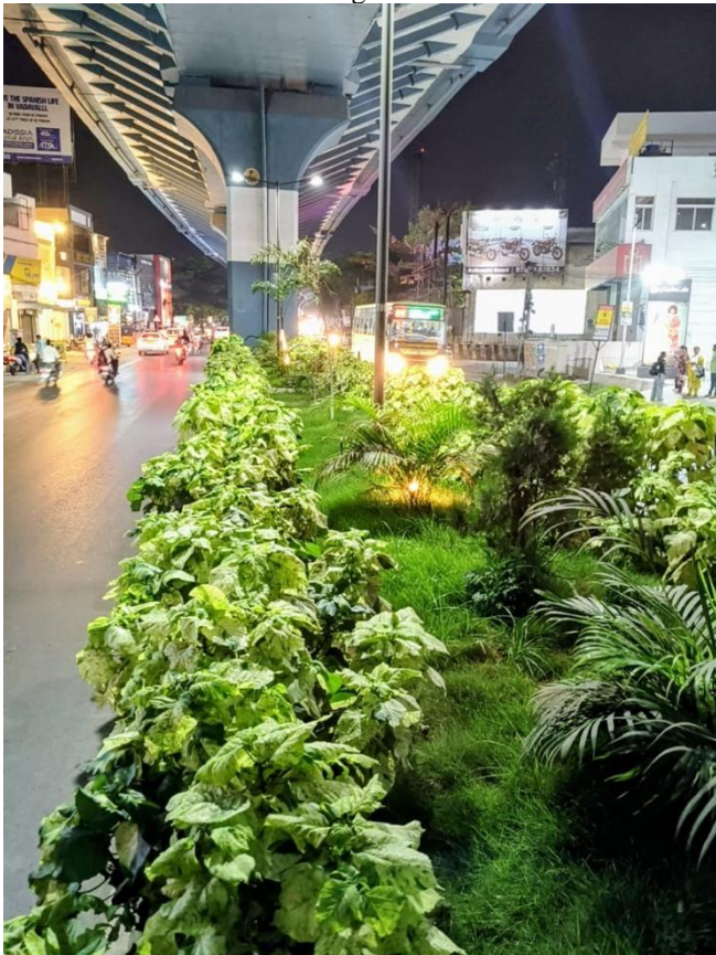
Fig 37. Edge Plantation between Pier Protection Wall
