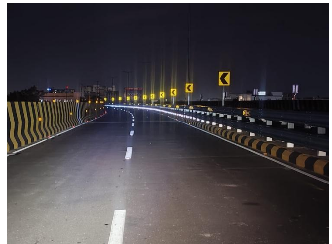
Fig 31. Reflective stickers on Crash Barrier Post.
