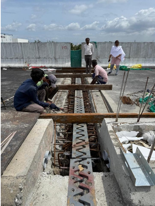
Fig 13. Sinus Plate Expansion Joint
