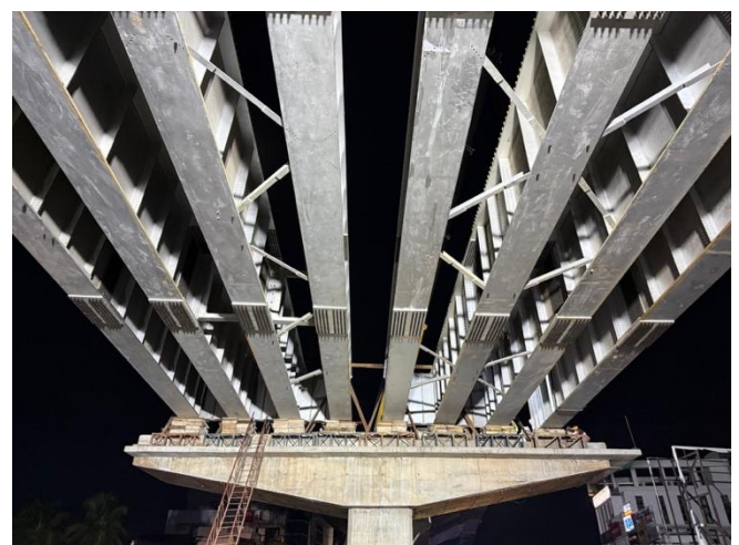
Fig 12. Launching of Steel Girders.
