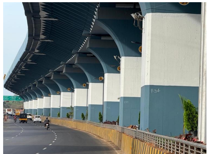
Fig 22. 6 Lane Atgrade Configuration.
