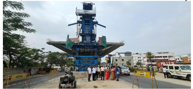
Fig 7. Segment Launcher.
