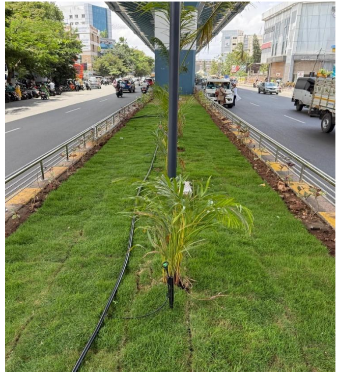
Fig 38. Green Grass Carpet between Pier Protection Wall
