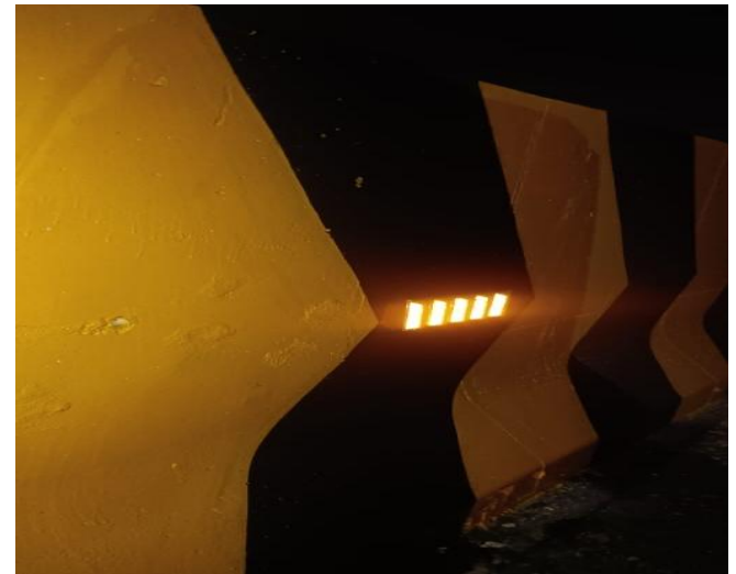
Fig 32 Megalux Reflective Panel over Crash Barrier
