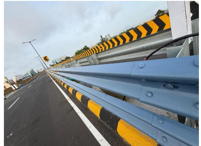
Fig 17. Metal Beam Crash Barrier
