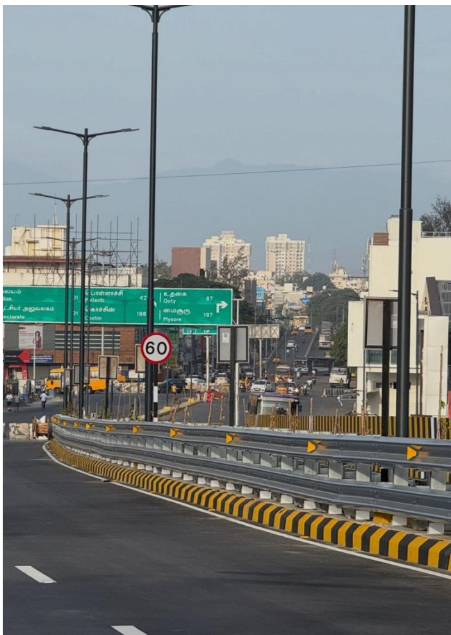
Fig 16. Continuous Centre Median in Elevated Corridor
