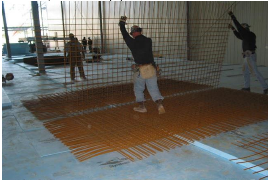
Figure 2. Structural WWR handling and placement in construction sites [14]
