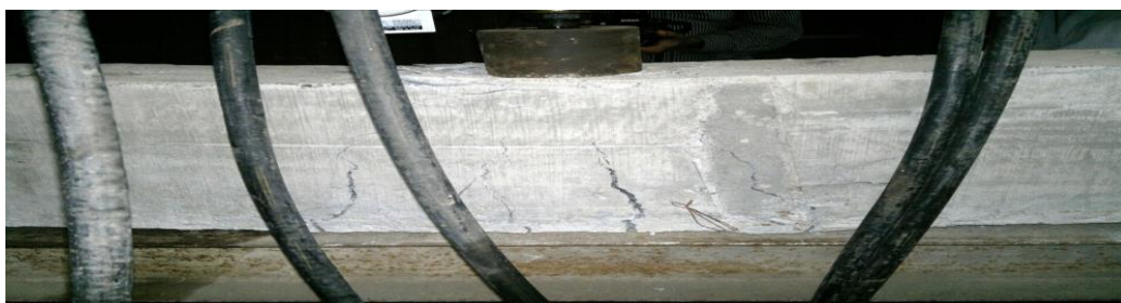
Figure 4.2. Flexural Crack in FC Beam
