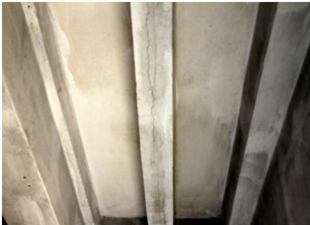
Figure 4.11. Crack Appeared in the Bottom of Ribs
