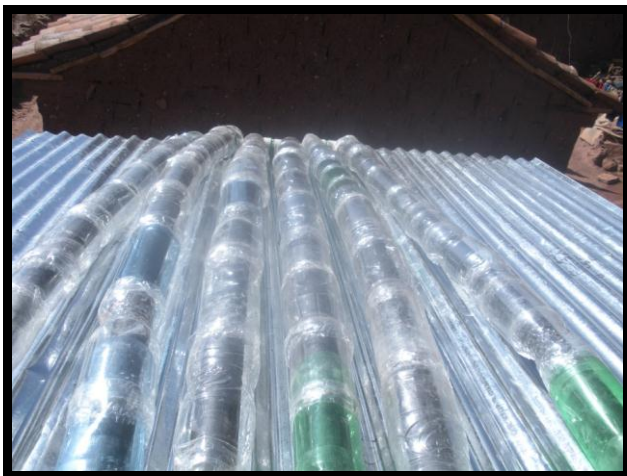
Figure 9. "Pipe-In-Bottle" configuration installed on each solar shower/latrine combo constructed in Pampoyo
