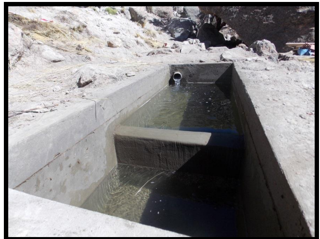
Figure 5. Working view of 6,000 L sedimentation basin constructed in Pampoyo
