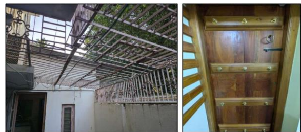
Fig. 4. Waste recovery through reuse of doors retrieved during renovation
