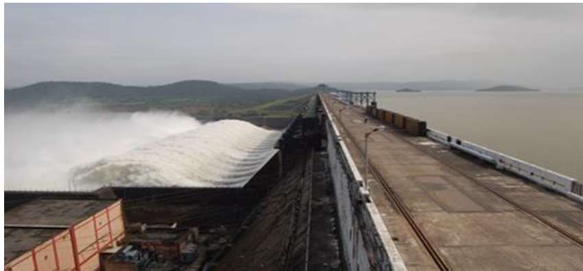
FIG.1. HYDRAULIC STRUCTURE (UKAI DAM)
