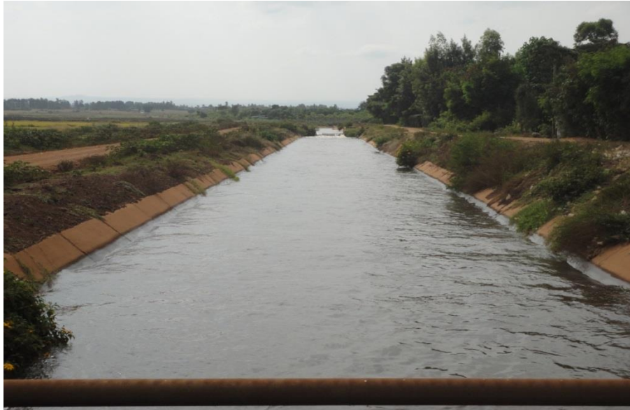
Figure 4: A section of lined trapezoidal Thiba Main Canal
