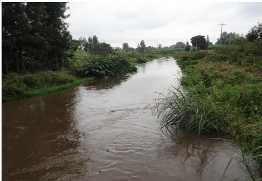
Figure 3: A section of Link canal II
