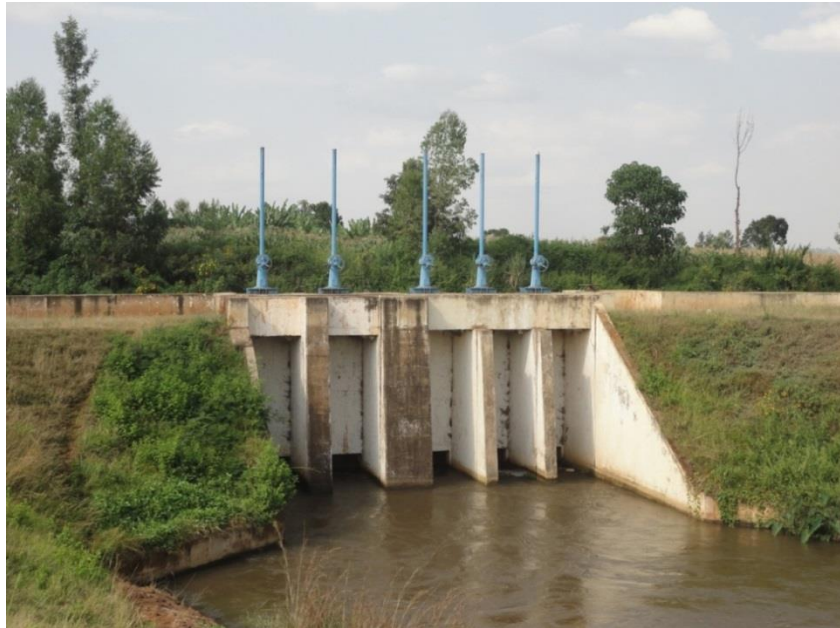
Figure 2: Upstream view of gates at Thiba off-take in MIS
