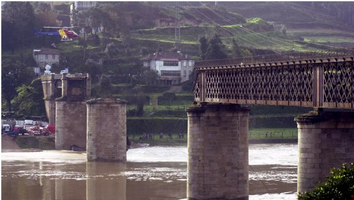
Figure 4 – Hintze Ribeiro Bridge with high flow after the pillar fell
