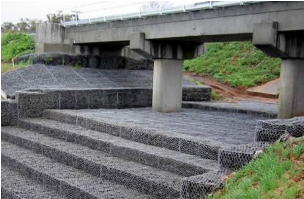
Figure 9– Example of application of gabion systems in the protection of bridge pillars ( https://www.mdpi.com/2673-4117/1/2/13 )
