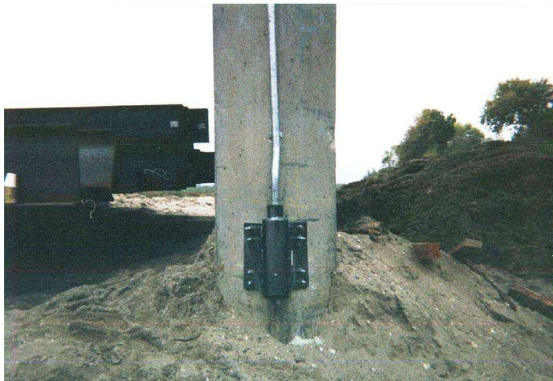
Figure 13 – Sonar placement on the upstream face of a bridge pier over the Salinas River in California, USA, to measure local erosion depths
