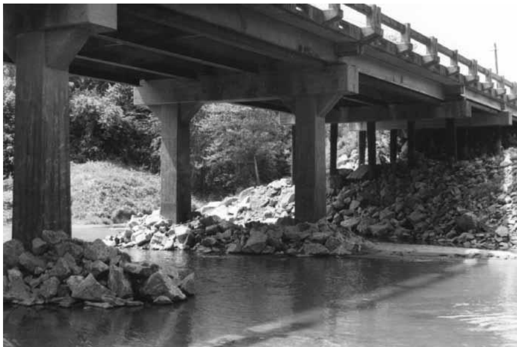
Figure 7 – Bridge pillars protected by natural rockfill. Pinhão Bridge (Portugal)
