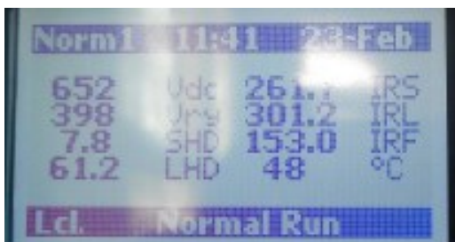
Fig 7.7 a Source Harmonic distortion – 7.8% at 76.5 % AHF rating ( 153 A)
