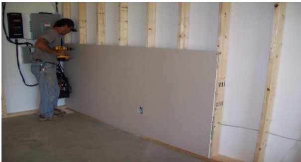
Fig. 3. Use of plasterboard sheet interior wall [1].
