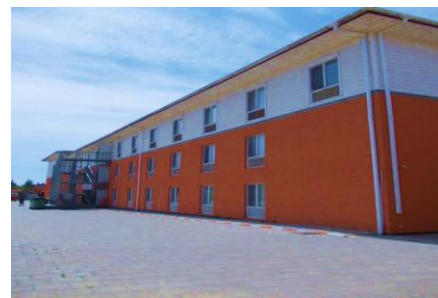
Figure.9.Longson Dormitory (Photo by author in 20th of April 2014)
