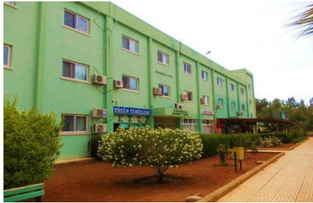
Figure. 11. Sanel Dormitory (photo by author in 18th of April 2014)
