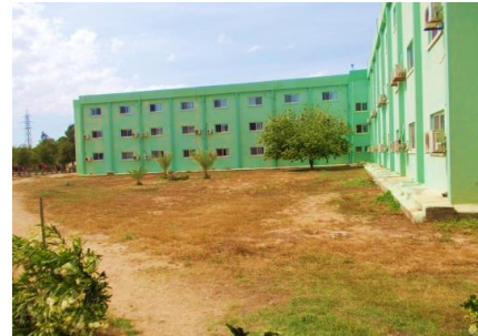
Figure 14. Sanel Dormitory (photo by author in 18th of April, 2014)
