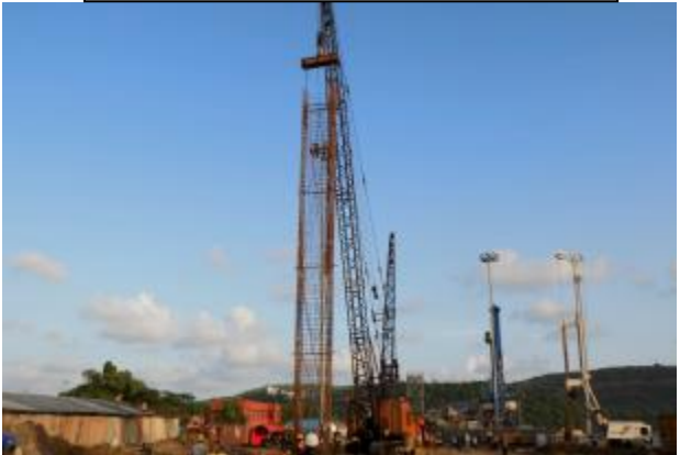
DIAPHRAGM WALL CAGE LOWERING INTO BORE HOLE
