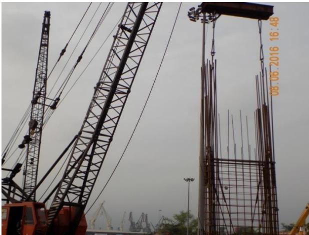
DIAPHRAGM WALL CAGE LOWERING INTO BORE HOLE
