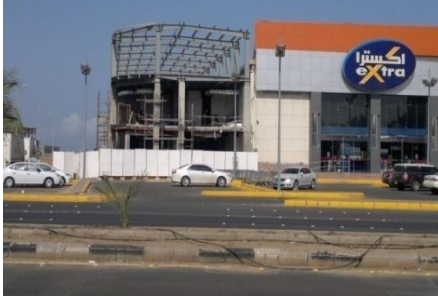
Picture (6) The future extension of the metal construction
