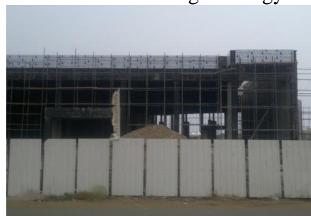
Picture (3) Isolation construction in compatible with the hot environment
