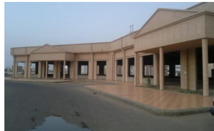
Picture (4 - a) Cover Metal established of abroad in accordance with the surrounding environment.
