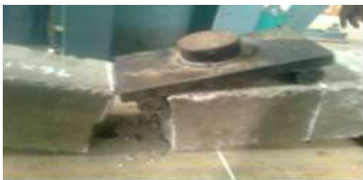
Figure 4 Failure of Beam Specimen at Flexural Load
