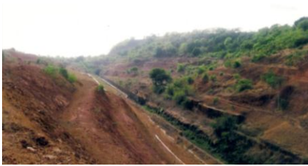
Fig. 1. Pomendi cutting before flattening of cutting slope
