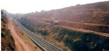
Fig. 2. Pomendi cutting after flattening of cutting slope during April 2011
