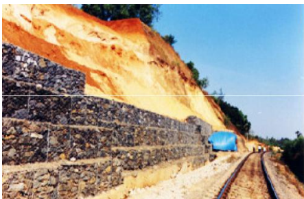
Fig. 4. Gabion constructed in problem area as solution
