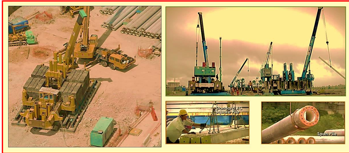
Figure33: Displaying the hydraulic Jack-in piling machines in construction site in Kuala Lumpur
