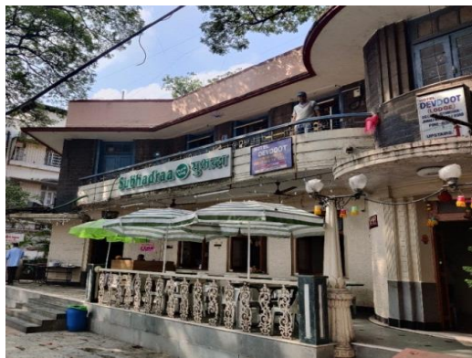
Fig.8. This structure is now a commercial building is a mix of vernacular style with stone masonry and plastered surfaces, and also has art deco influence seen in curved balconies, horizontal lines, metal railings, and grills for balcony.
