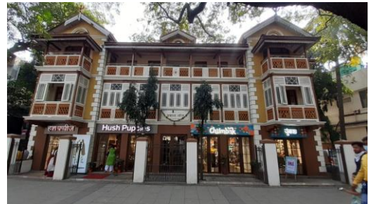
Fig. 6. It is a modern vernacular building with a central balcony and two projecting balconies. Art deco influences cement color and decoration, portholes. A traditional element like gabled roofs and balcony grills, and louvered ventilators.
