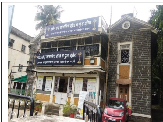
Fig.5. This residential structure, now used for commercial activity, is load bearing with rectangular stone facades and triangular pedimented roofs borrowed from traditional vernacular style: the portholes, colored concrete strips, and metal grill windows showing art deco influence.
