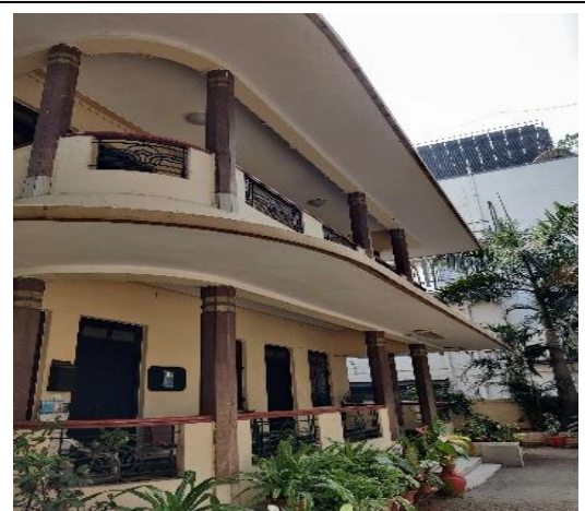
Fig .7. Art deco style with curved chajja, metal grills for balcony and windows. Rounded corners, concrete, and stucco painted in pastel colors, horizontal bands, flat roof, etc.
