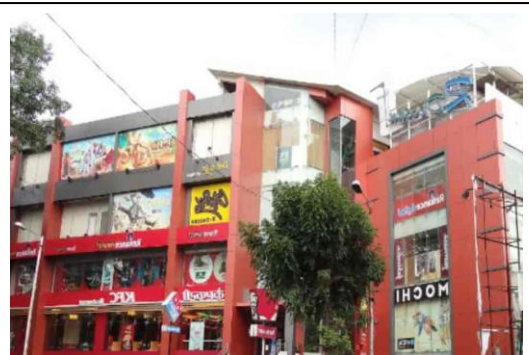
Fig.11. Contemporary modern, RCC structure with glass and alucobond panel cladding on external facades
