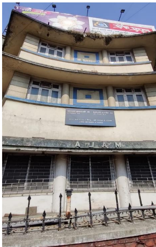
Fig. 9. Art deco style with curved chajja, metal grills for balcony and windows. Rounded corners, concrete and stucco painted in pastel colors, horizontal bands, flat roof, etc.
