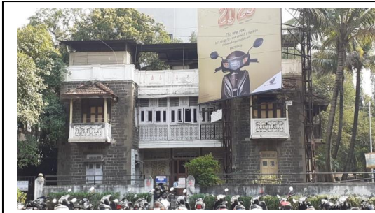
Fig.3. This residential structure is a hybrid of many styles showing projecting balconies with metal railings. A central staircase stands out with art deco-styled metal grills for staircase block and renaissance pediment and a combination of ashlar and rusticated stone masonry.
