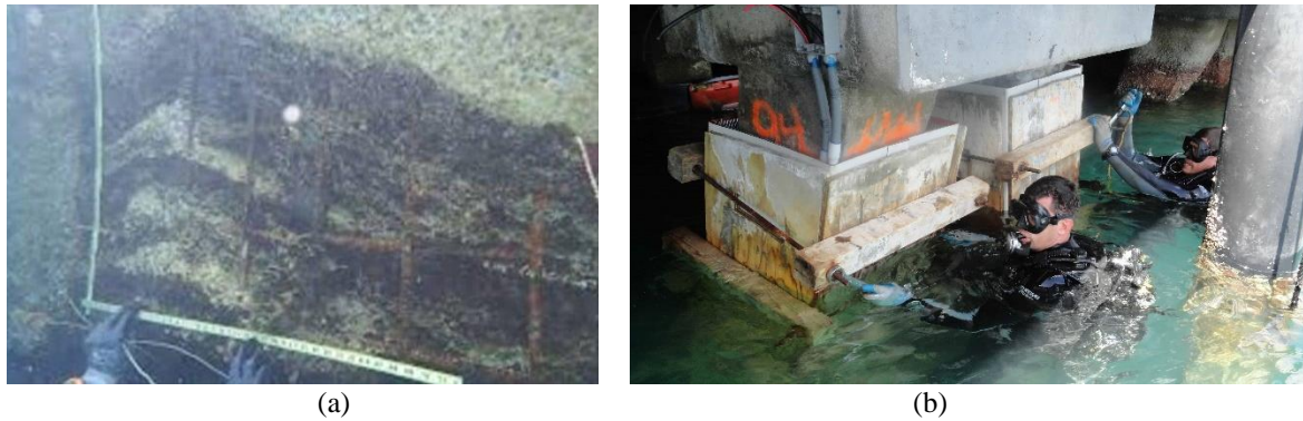
Fig. 3. Bridge showing (a) exposed reinforcement in pile (b) divers inspecting for cracks underwater
