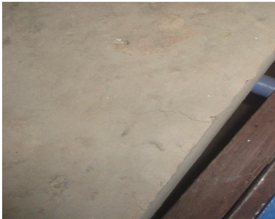
Fig. 3.15: Cracks formed in the specimens after treated to 600°C
