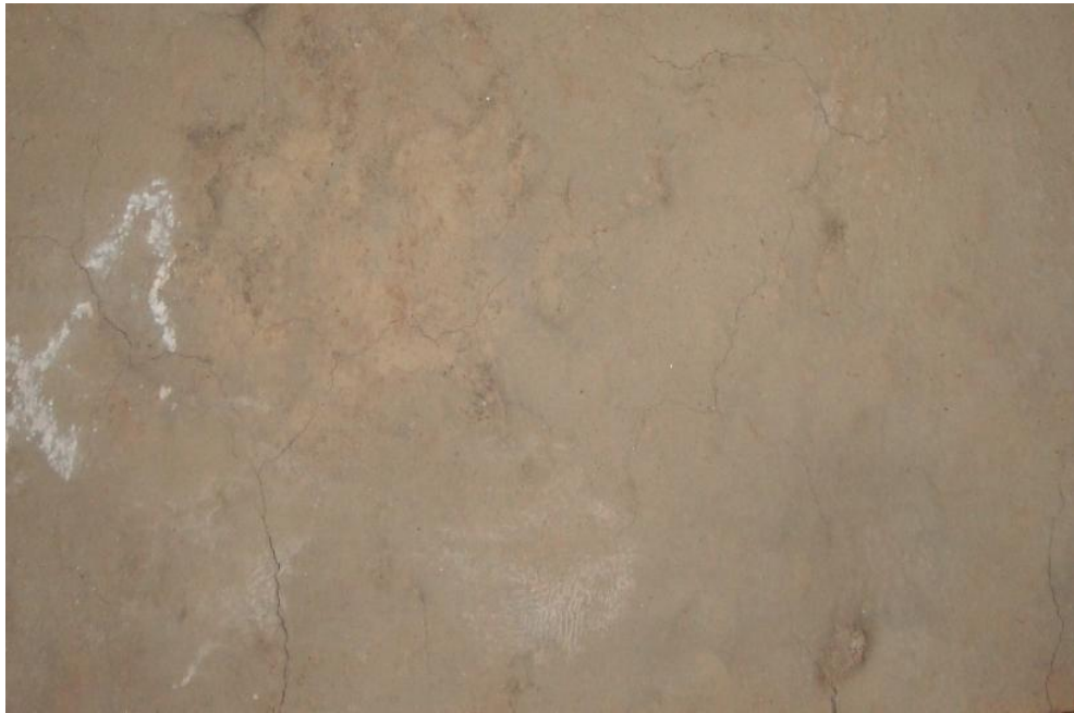
Fig. 3.16: Cracks formed in the specimen after treated to 800°C
