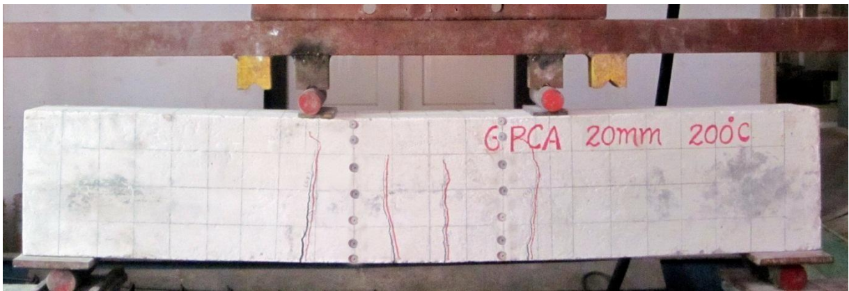
Fig. 4.18: Crack pattern of GPCA 20mm 200°C
