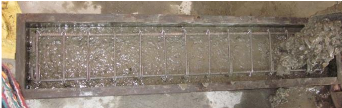
Fig. 3.5: Casting of GPC 20mm beam specimen
