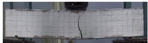
Fig. 7. Flexural failure of the series #2 beam
