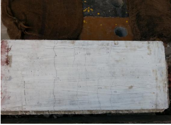
Fig 3: Crack pattern on the surface
