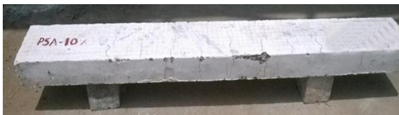
Fig. 21 Crack Pattern of GPC 10 % Sun Light Cured Specimen.
