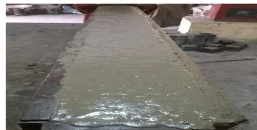
Fig. 2 Casting of GPC in Beam Mould
