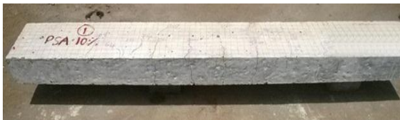
Fig. 19 Crack Pattern of GPC 10 % Oven Cured Specimen.
