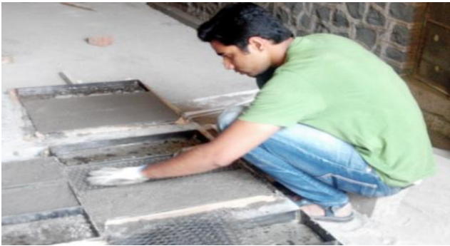
Fig 7-Placing of mesh layers in mortar
