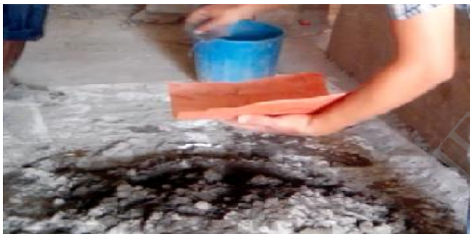
Fig 2-Mixing of steel fibers in mortar
