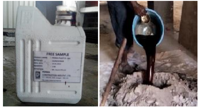
Fig 4-Admixture (Perma PC202) after mixing with water used in mix
