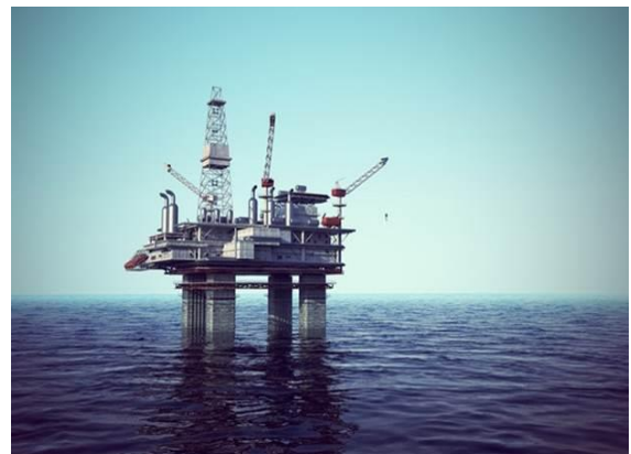
Fire ice extraction plant (small scale)
