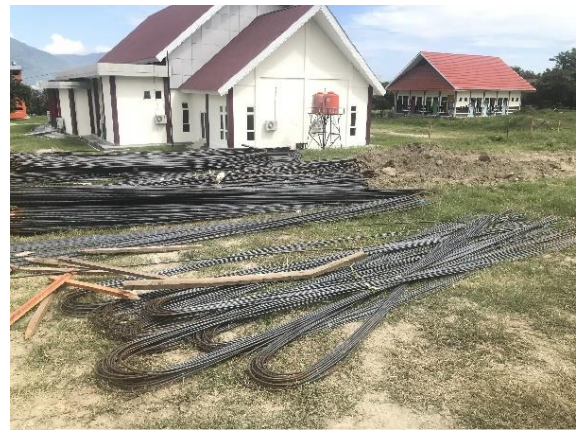
Figure 6. Stock Iron material on site
