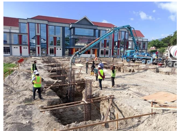
Fig 2. Casting pedestal column with competent labor.
