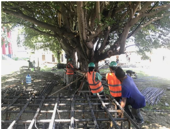
Fig 4. Reinforcing footplat
