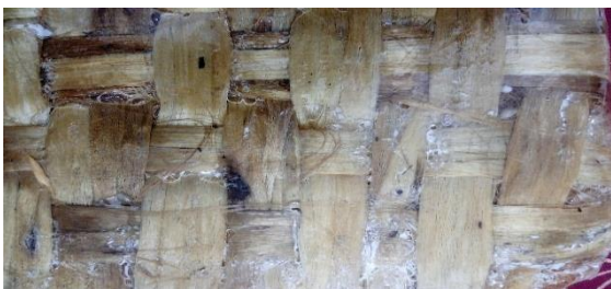
Figure 3.7 Uneven Surface on Composite
