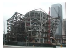
Figure 1 Internal Lattice Frame
