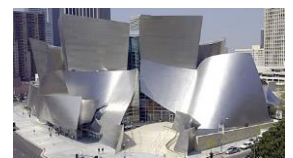
Figure 2 Metal sheet of doubly curved surfaces
