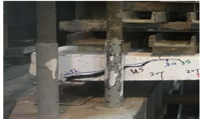
Figure 17: Shear cracks of specimen (0.06%-U)
