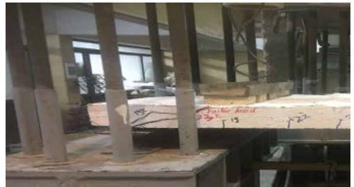
Figure 21: Shear cracks of specimen (0.1%-O)
