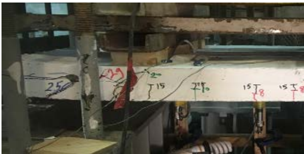
Figure 23: Shear cracks of specimen (0.06%-T)
