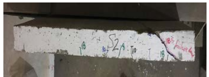
Figure 13: Shear cracks of specimen (R-N-O)
