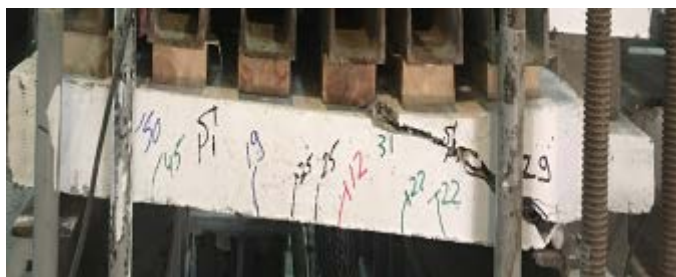
Figure 11: Shear failure of specimen (R-N-U)
