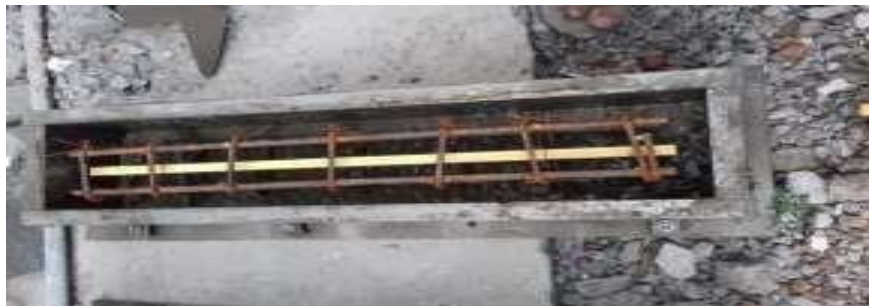
Fig -4: Casting of I-section GFRP beam
