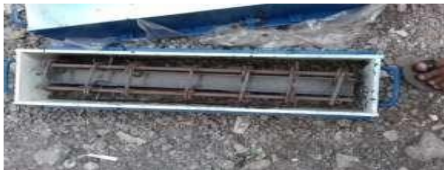
Fig -5: Casting of C-Channel GFRP beam
