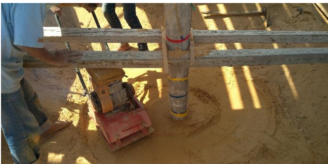
Fig. [13] Placing Compacted Soil around Tested Pile for group (1) – Single Pile
