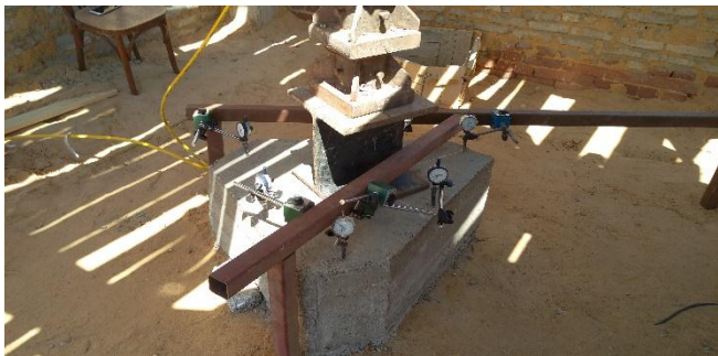
Fig. [20] Loading Jack and Dial Gauges Setup for Group (3) – Group of Three Piles
