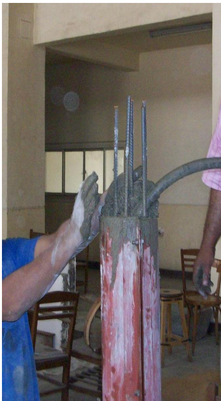
Fig. [7] Casting of Piles
