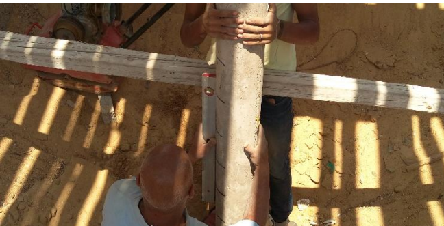
Fig. [12] Vertical Alignment of the Pile for Group (1) – Single Pile
