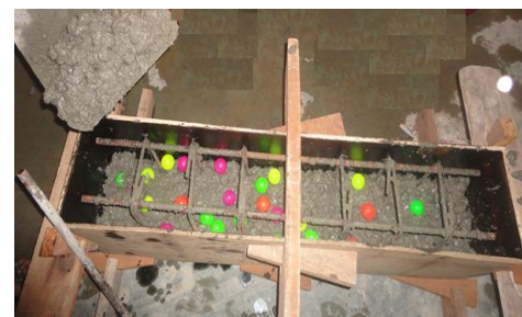
Fig.3. Casting of Replaced Beam
