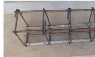
Fig.1. Reinforcement Cage for Beam Specimens
