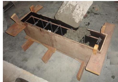
Fig.2. Casting of Control Beam
