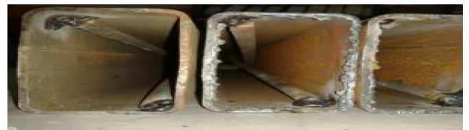
Fig. 2 Welding of Shear Connection
