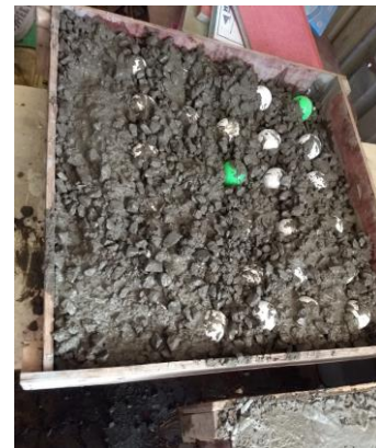
Fig-4: Concreting of Bubble deck flat slab
