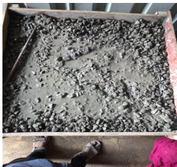
Fig-2: Concreting of conventional slab
