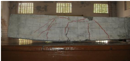
Figure : 6 – Crack pattern of Beam
